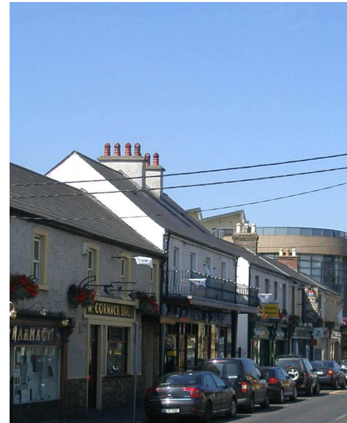
Fig 12.12 Typical Street View and Illustration of existing accumulated clutter.
