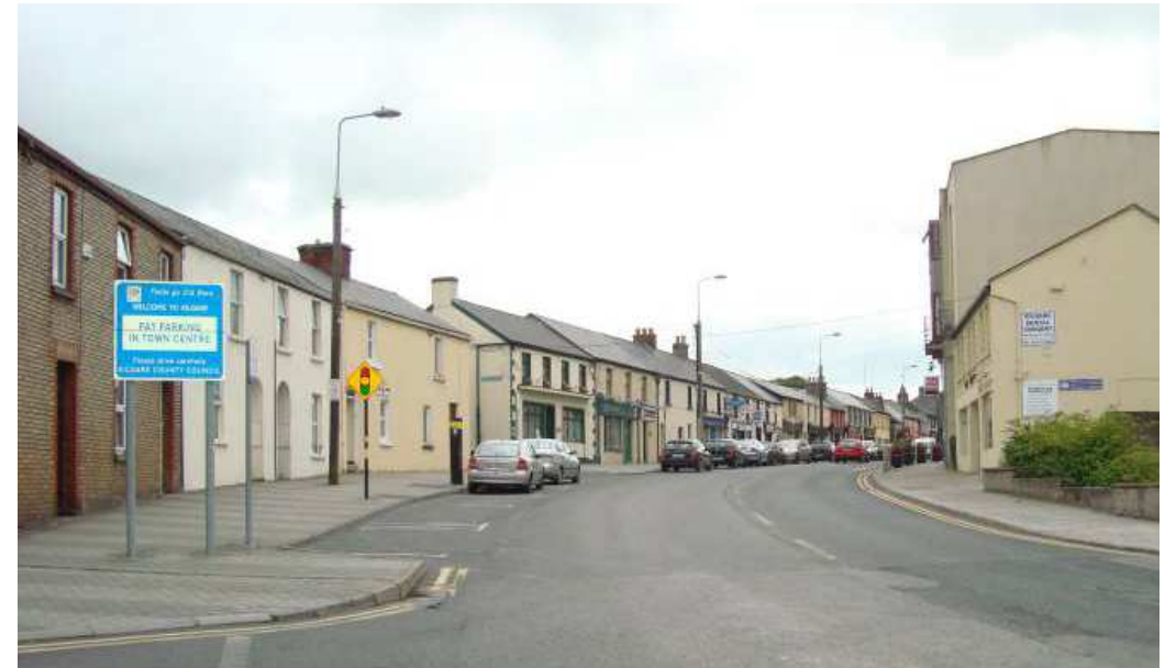
Fig. 7.18_Claregate Street From Cleamore Road Junction
