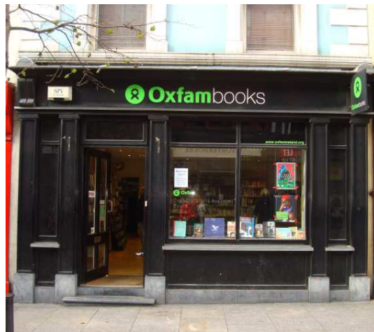
Fig 12.6 Oxfam Parliament Street, Dublin Example of Contemporary shop front in traditional style, representing an appropriate approach for potential replacement of modern shop fronts such as on Market Square.
