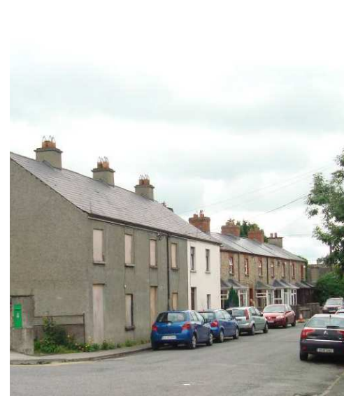
Fig. 7.38_Cleamore Road from Claregate St.
