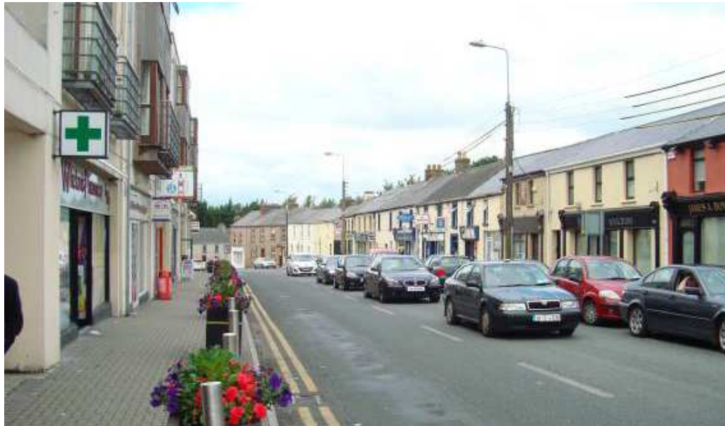
Fig. 7.16_Claregate Street From Mid Way Along Street, View Westwards
