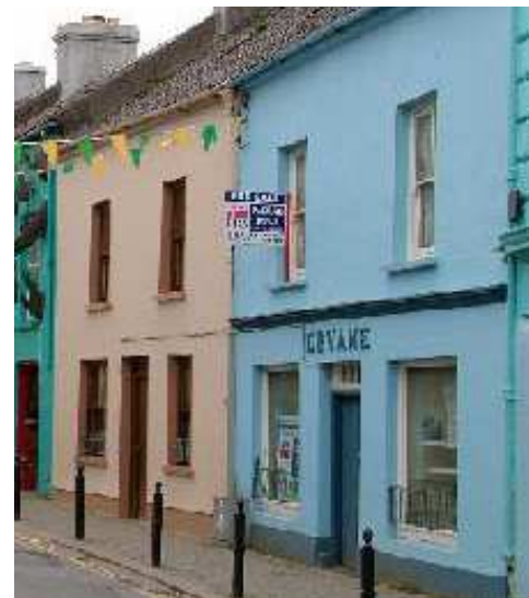
Fig 12.8 Examples of Modest shop front approach in Dingle Co. Kerry, utilising window and door openings positioned with consideration to the existing first floor windows, and their proportions, with simple signage demarcating the commercial activity. This example is an appropriate approach for commercial uses on the northern side, and at the western end of Claregate Street.
