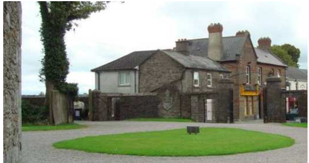
Fig. 7.9_Entrance Forecourt To Cathedral
