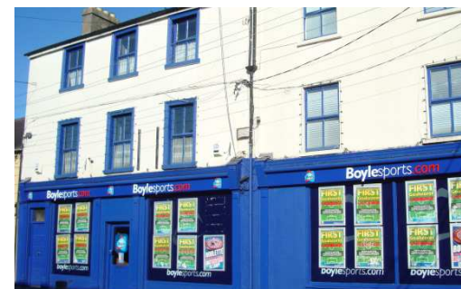
Fig 12.9 Inappropriate - Example of Negative Impact of Signage Placed on Location of Original Shop Fronts
